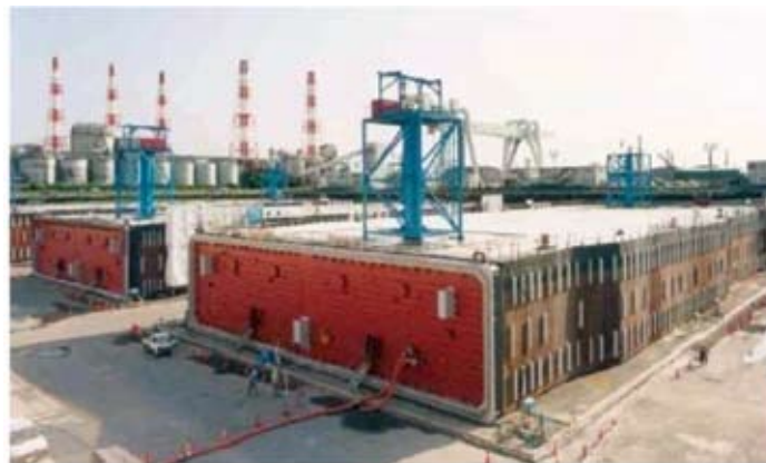
Fig.(13) Sandwich structure applied to immersed tunnel in Kobe, Japan[7]
