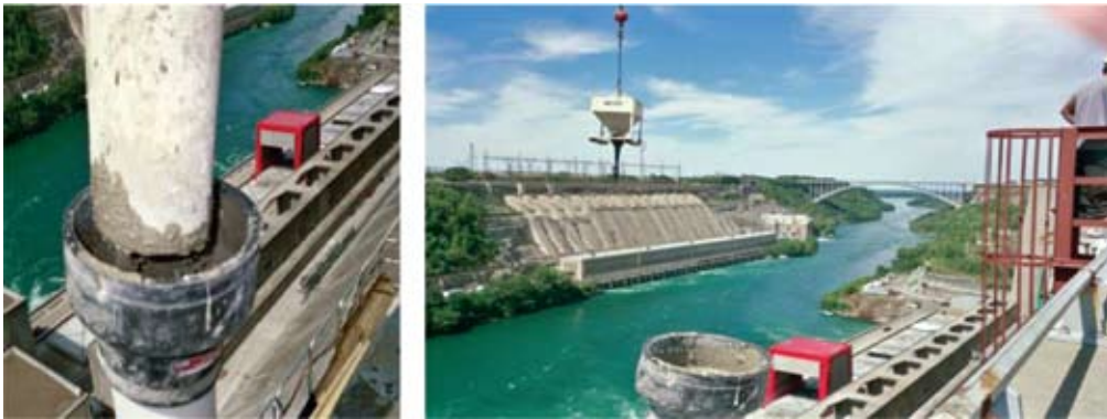
Fig.(16) View of the Robert Moses Dam
